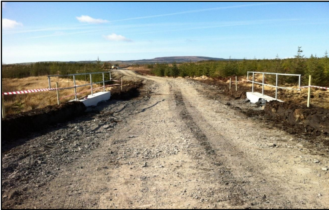
Figure 3-17 Dirty water containment at watercourse crossings
