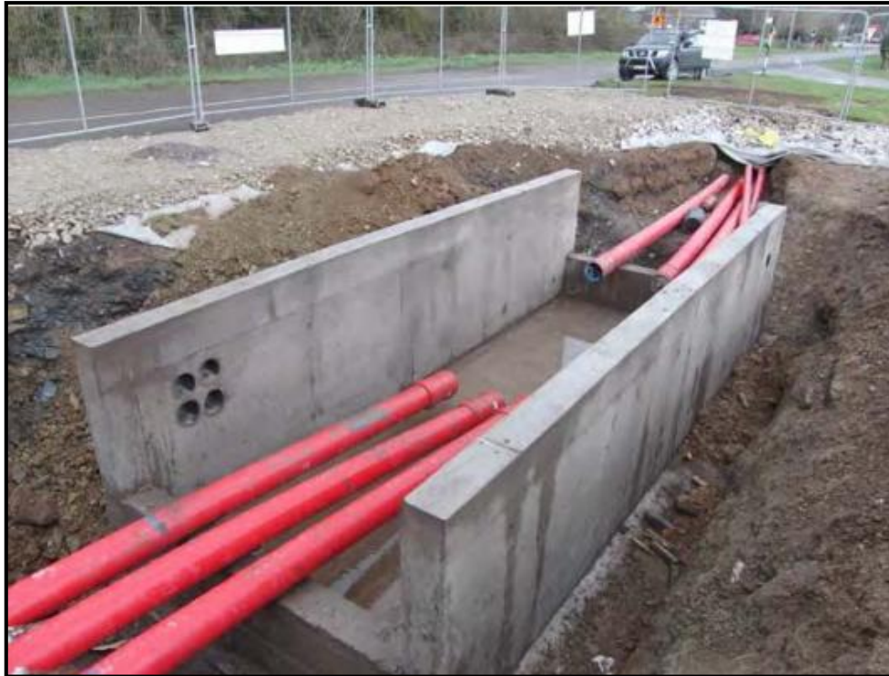
Figure 3-14 Typical joint bay construction
