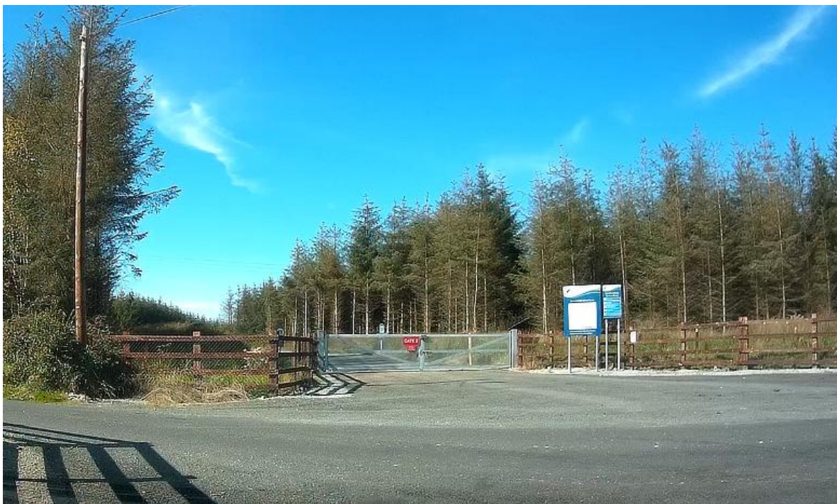
Figure 3-1 Typical Wind Farm Entrance
