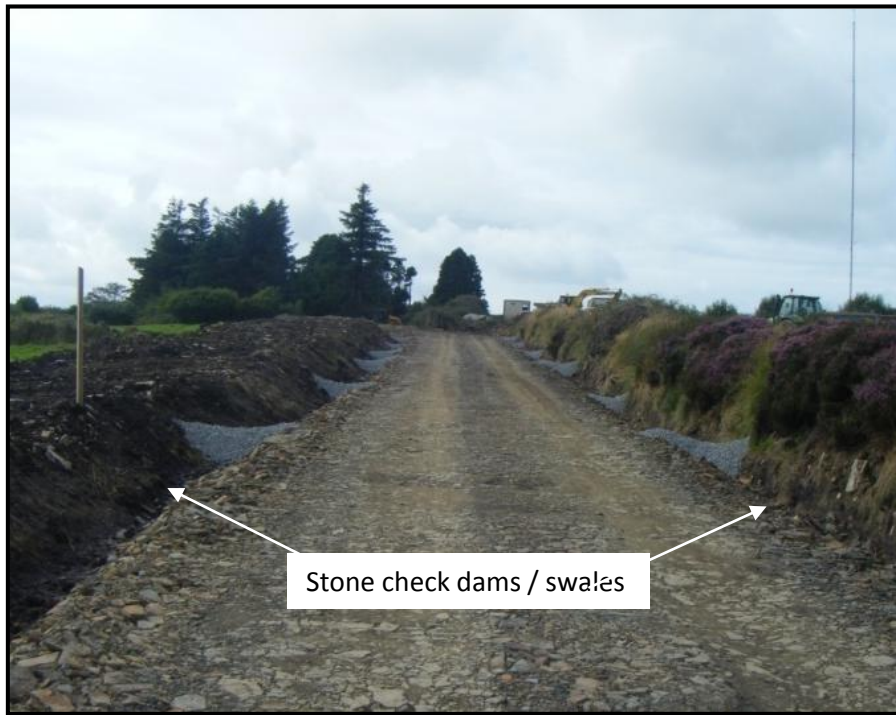
Figure 3-30 Examples of check dams along roadside drainage channels
