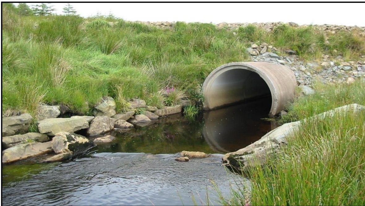
Figure 3-16 Typical drainage channel crossing
