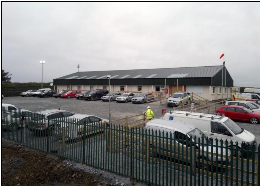
Figure 3-27 Typical temporary site construction compound on a wind farm
