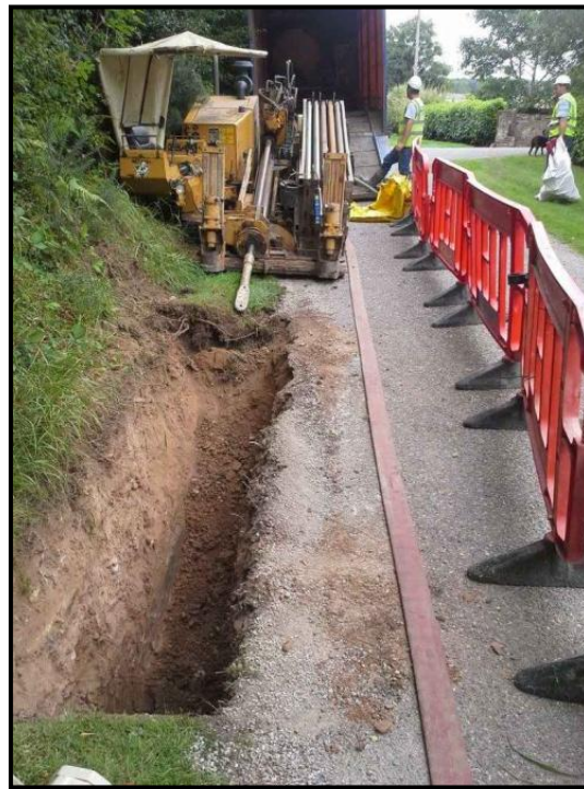
Figure 3-24 Typical directional drilling rig and launch pit
