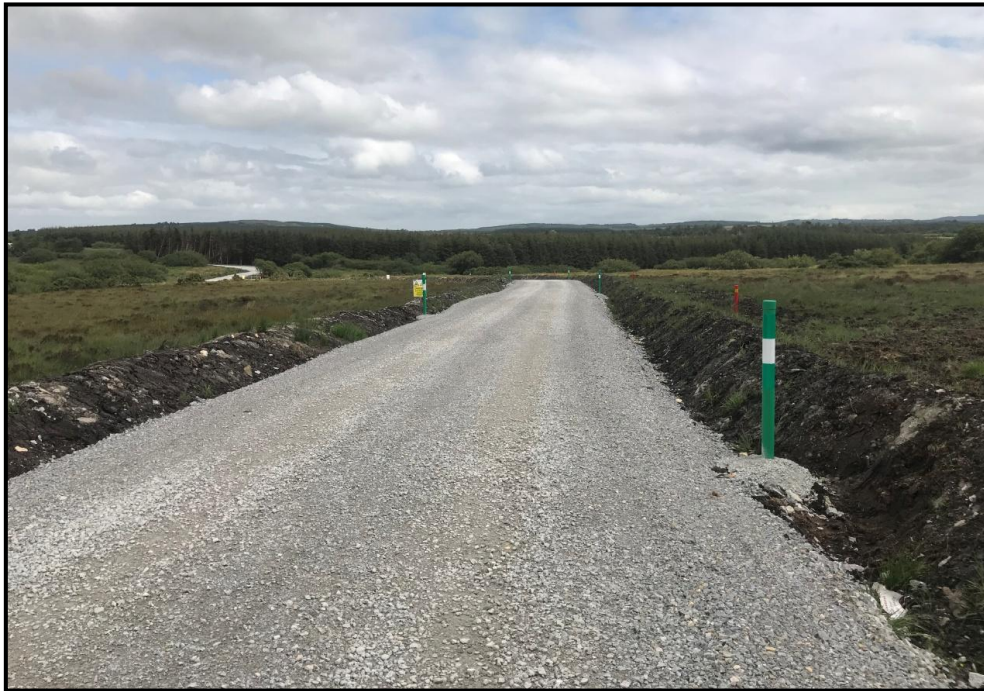
Figure 3-6 Typical floated road on a wind farm
