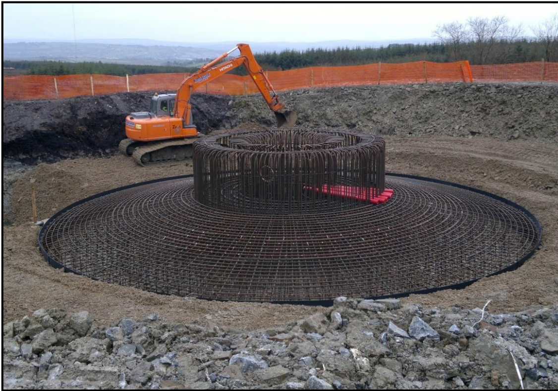
Figure 3-9 Typical construction of a wind turbine base
