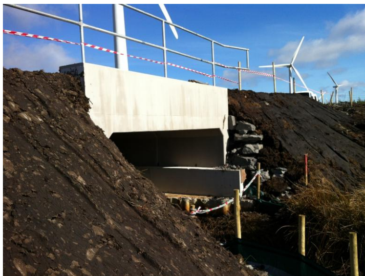
Figure 3-15 Typical Rectangular Box Bottomless Culvert
