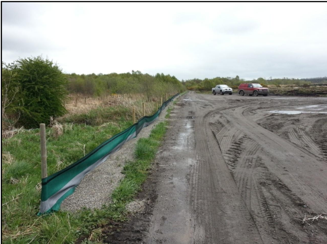
Figure 3-18 Silt curtain containment along existing roads near watercourses
